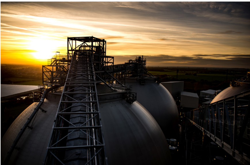
Four biomass domes at Drax can store 75 kt pellets each and supply also the high demand in winter.
